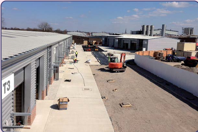
Twenty-one industrial units at the Leyton Industrial Village, London.
