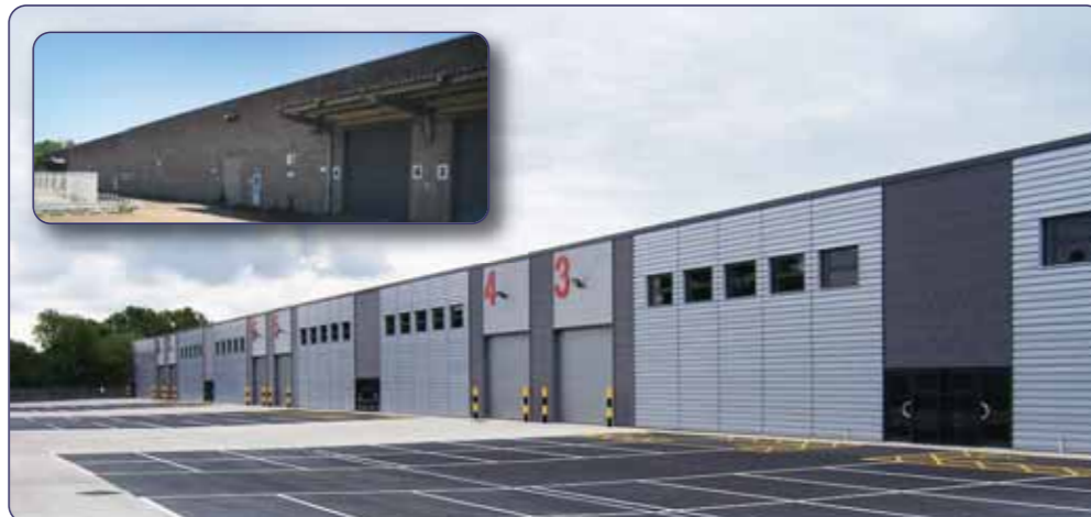
HIGH QUALITY: The site before Faircloth got to work in Amersham (inset) and the end result
